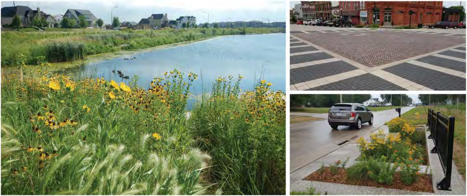
This pond is part of a series of natural treatment areas for stormwater. It was designed using the unified sizing criteria and it creates an open, park-like setting for residents to enjoy. Permeable pavers (top) and bioretention cells (bottom) also soak in rainfall and manage stormwater where it falls instead of shedding polluted water.
