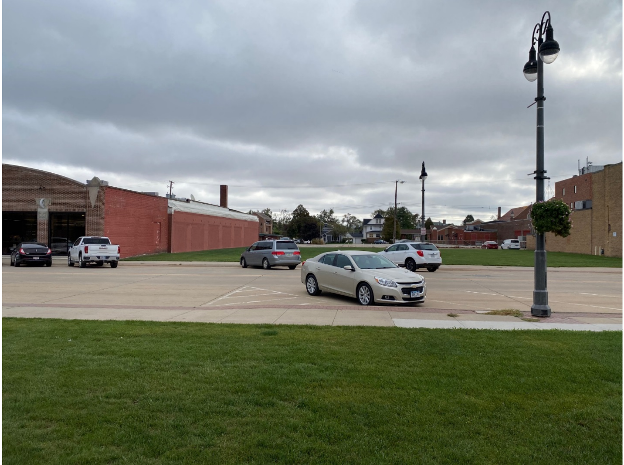
Photo of the demolition/cleared site of the former Grinnell Sporting Goods which relocated south on Main Street. This site is immediately east of the former McNally's site. The demolition makes way for a new multi-use building at this site. Grinnell College acquired this property in 2019. Development of this project is in process and construction is anticipated for spring 2022. 09/28/20
