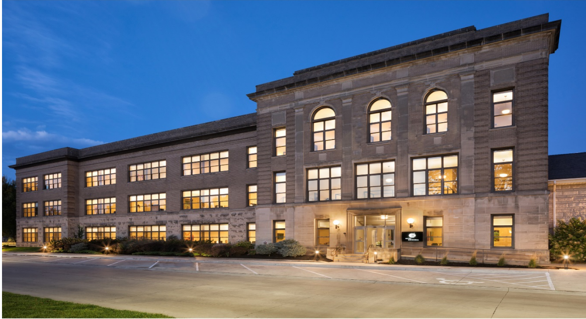
Photo of Hotel Grinnell East Façade in evening. This photo shows the conversion of the former Grinnell Junior High School into a boutique hotel-events center. 9/11/17
