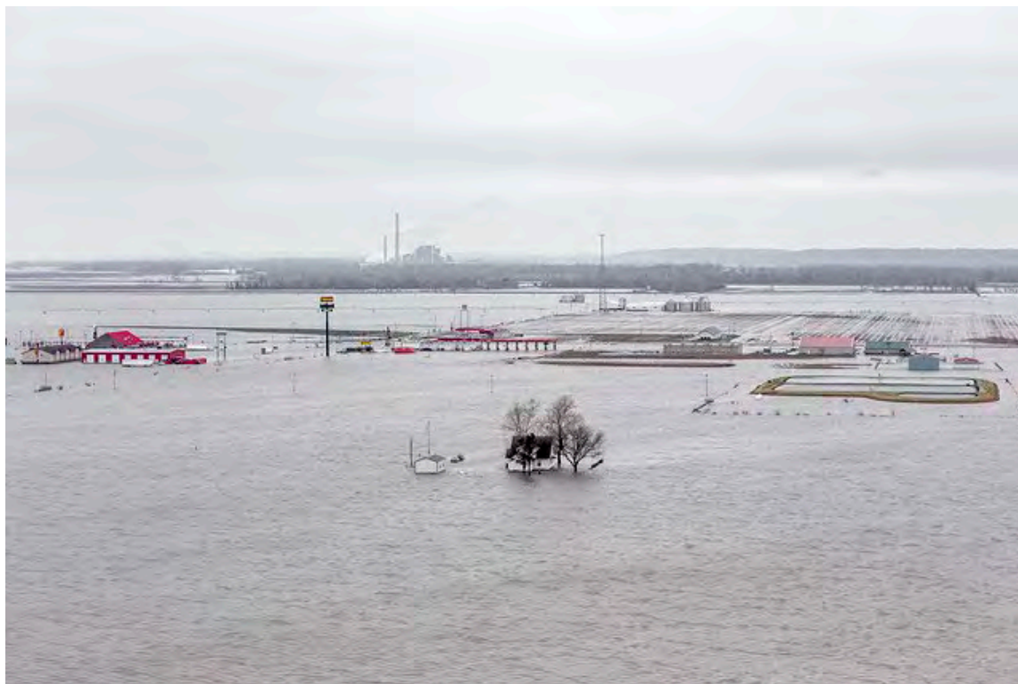
March 28, 2019 – I-29 & US 34 Interchange, Iowa DOT
