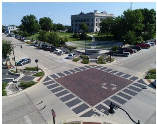
Example of stormwater bumpout intersection
